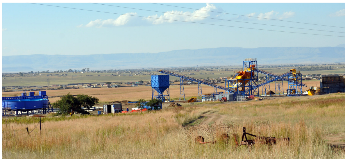
Picture of the Newcastle Project wash plant at site – 11 th April 2012
